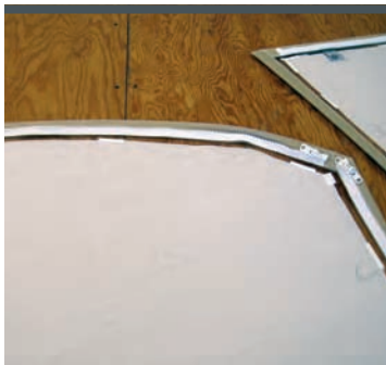
13 The panel with its zippers installed. The top zipper faces outboard to hide it.
